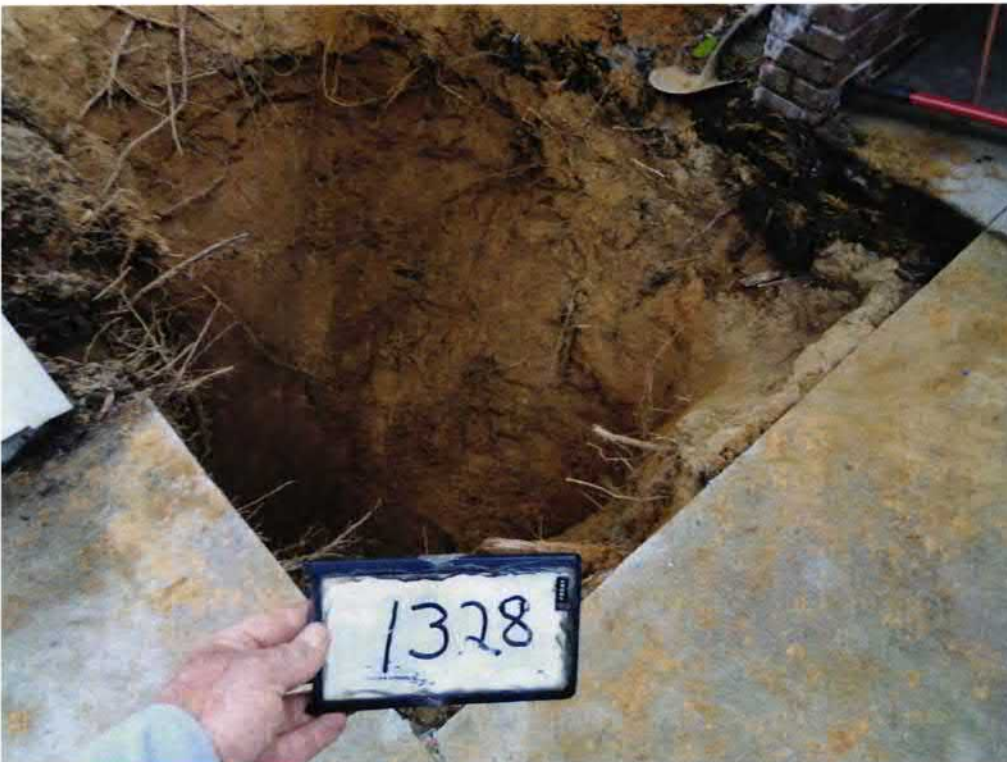
Picture 2: UST 1328Albatross excavation.
